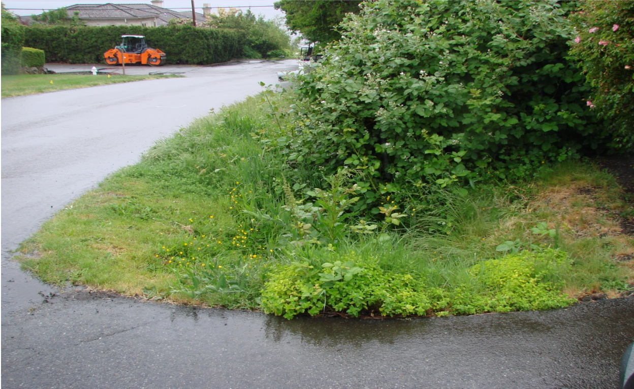
Photo #8 – Open roadside ditch on north side of SE 28 th Street – viewing west
