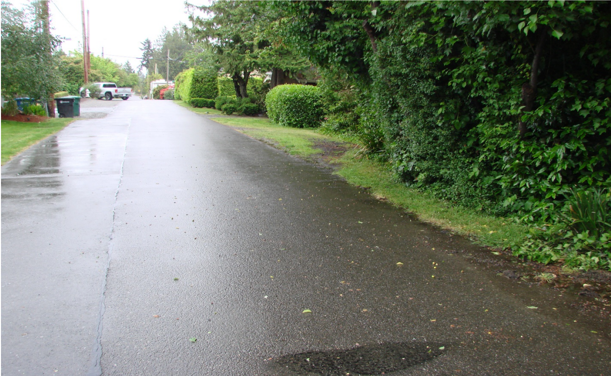
Photo #3 – Frontage along 61 st Avenue SE – viewing south (subject property to right)
